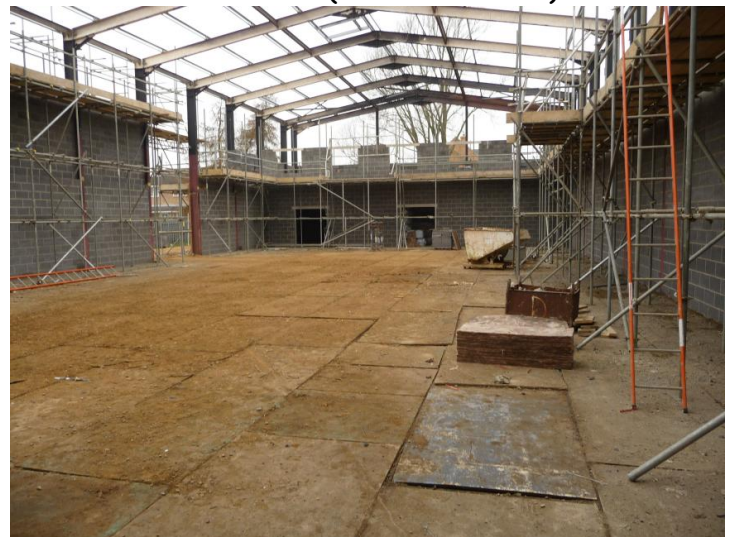
A view of the Main Hall.
