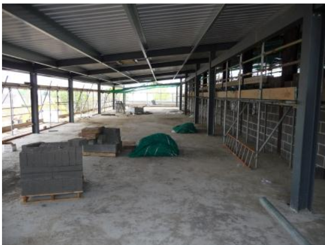
Archery range floor down and roof on.
