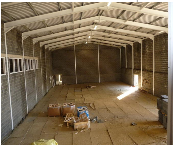
The steelwork in the hall has been painted.
